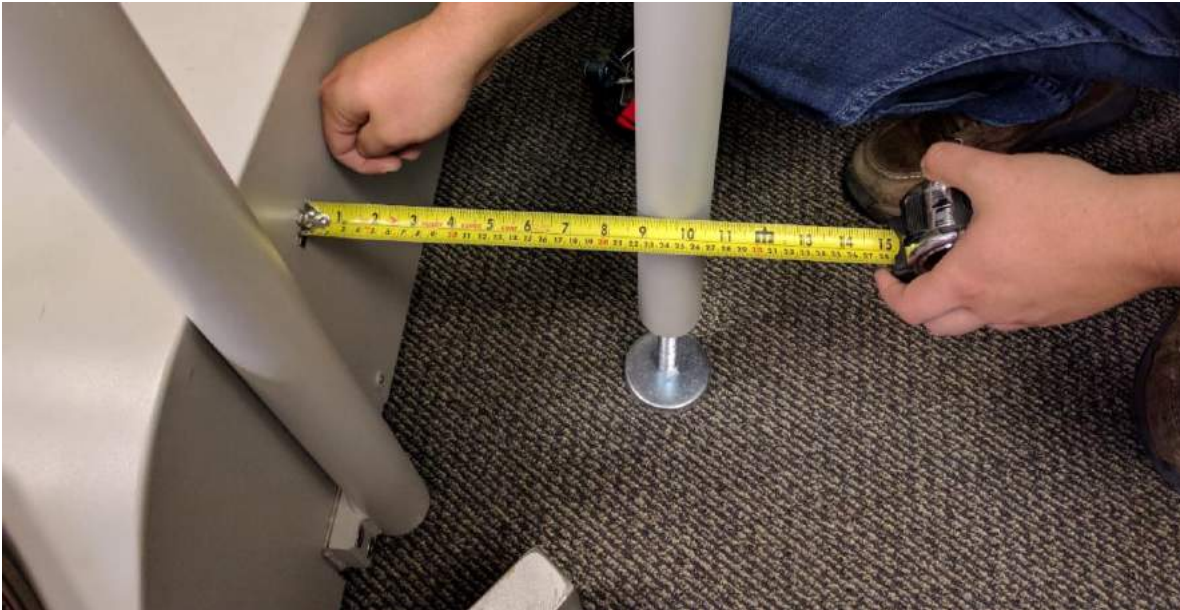
Figure 37 - Measurement from side of base to center of overhead structure post
