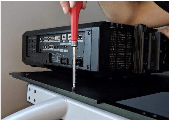
Figure 44 - Securing projector assembly to mounting rails
