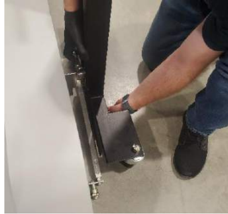
Figure 11- Lifting gate on bushing
