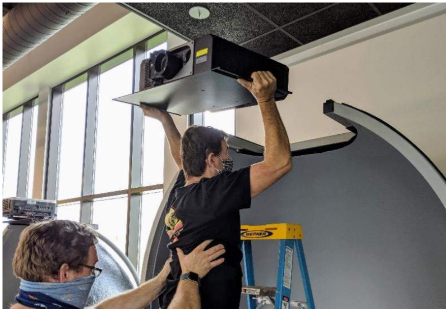
Figure 41 - Placing Projector assembly onto screen frame
